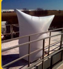
VZ Environmental introduced **VSoxz™** to minimize and contain airborne dust particles released from open batches on sand
